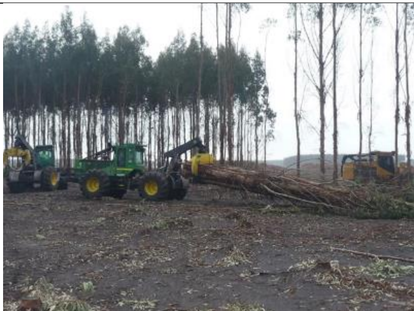
Figure 11: A skidder moving bunches of felled hardwood trees to a mobile chipper (Photo by DJ Geddes®)
